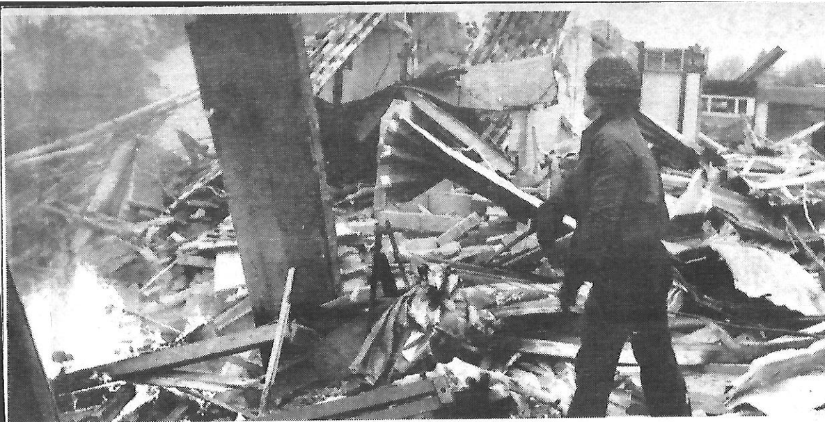
Demolition worker Col McDonagh feeds more debris to the flames
