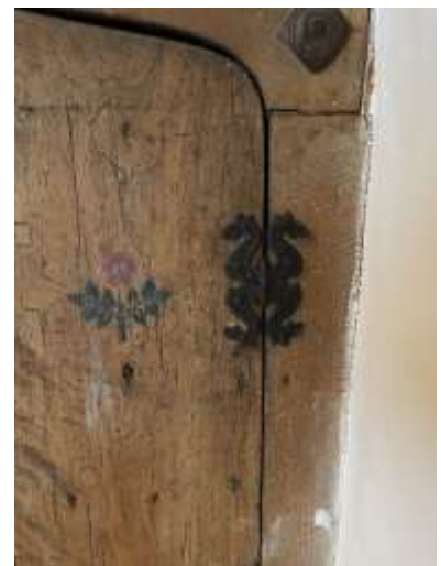
Figure 6: H-hinge on 'old' cupboard door
