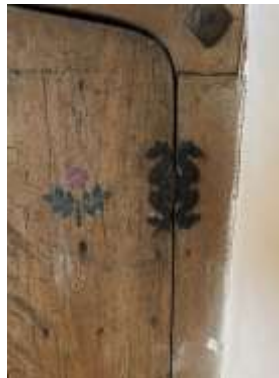
Figure 6: H-hinge on 'old' cupboard door
